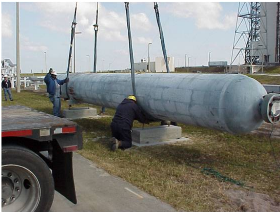
LC-37 Pressure Vessel Installation
