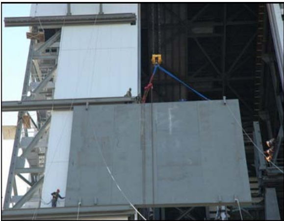
Photo: Pat Corkery/Lockheed Martin SLC-41 VIF Door Emergency Replacement
